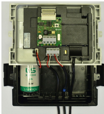
Picture 5.2 - Module installed in meter
